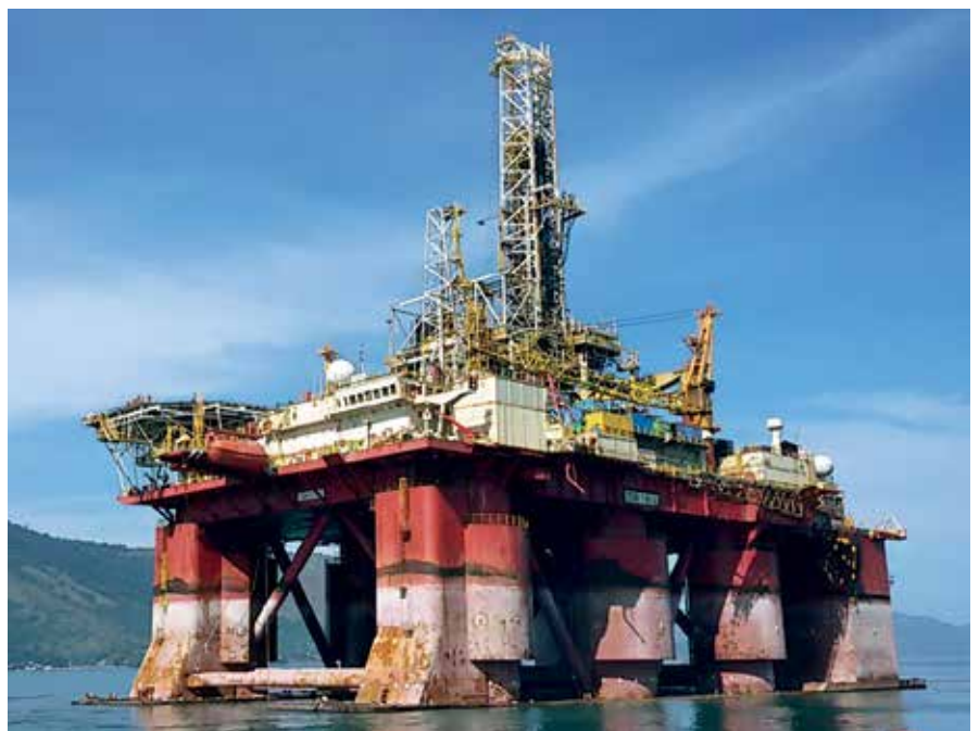
BrasFELS received the repair project semisubmersible ODN Tay IV on 7 July 2015
