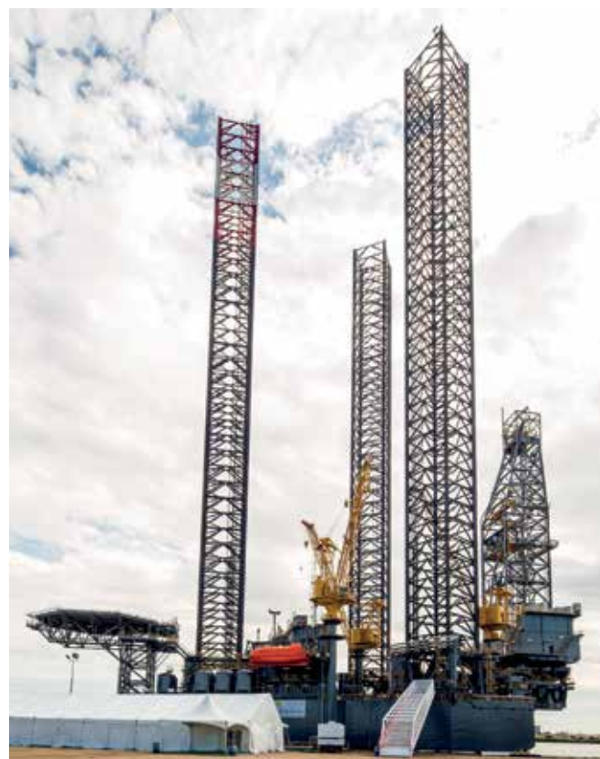
Keppel O&M has the expertise to build rigs of the LETOURNEAU™ design having previously completed 16 such rigs, including the COATZACOALCOS, a LETOURNEAU™ Super 116E design, which was built by Keppel AmFELS in Brownsville, USA
