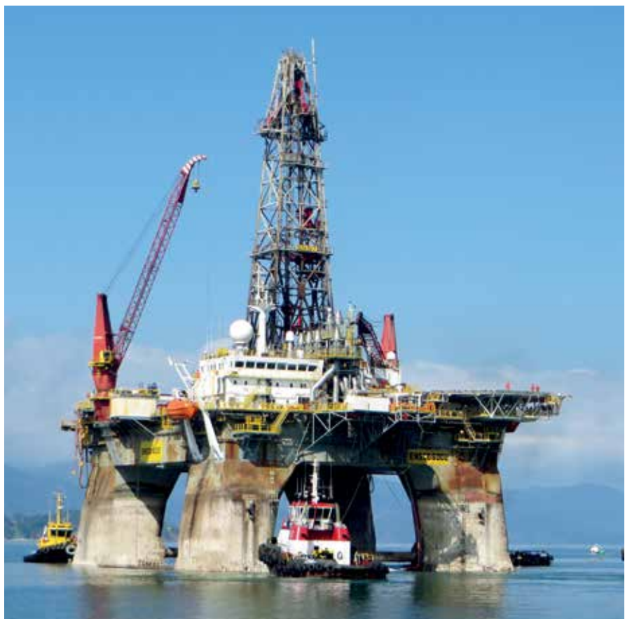
ENSCO 6002 leaving the shipyard on 29 July 2015 after successful repair works
